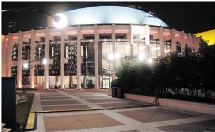
The main building in the Place des Arts complex, Salle Wilfrid-Pelletier is the largest performance hall in Québec.
